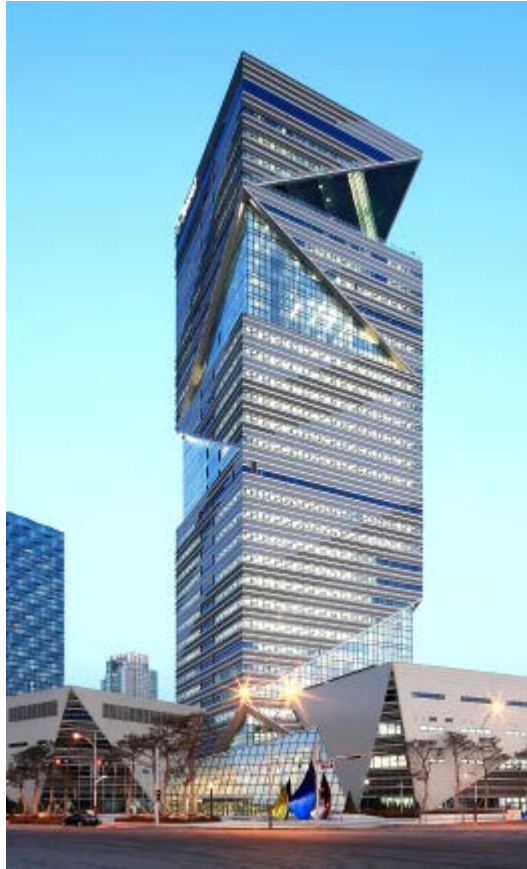
GCF Headquarters G- Tower, Songdo (South Korea)
